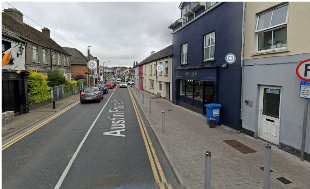
Figure 3-5 R392 (Looking West)
